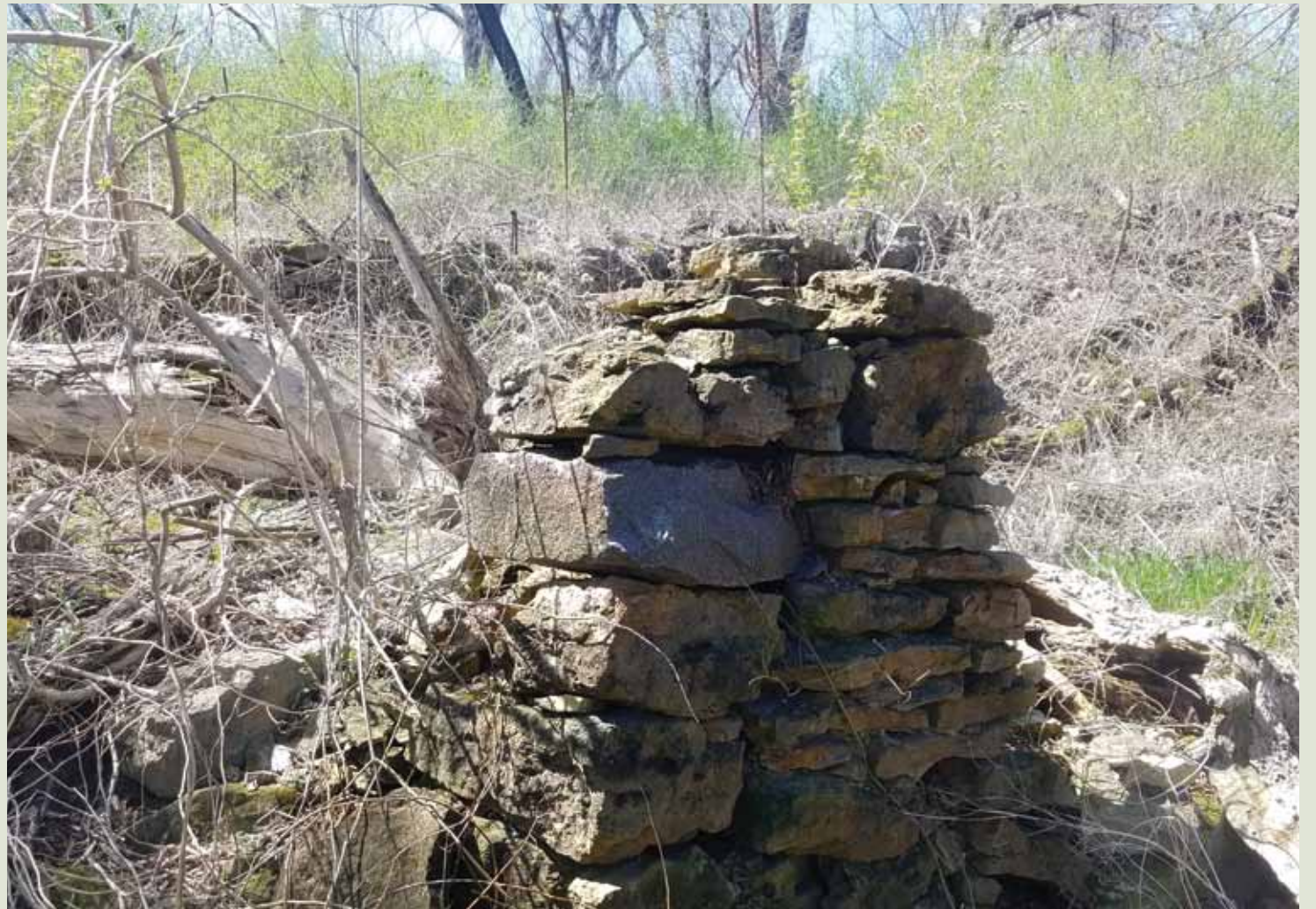
A REMENANT OF THE HISTORIC MILL RUINS ALONG EAGLE CREEK, POTENTIALLY BECOMING A STATE ARCHEOLOGICAL SITE.
