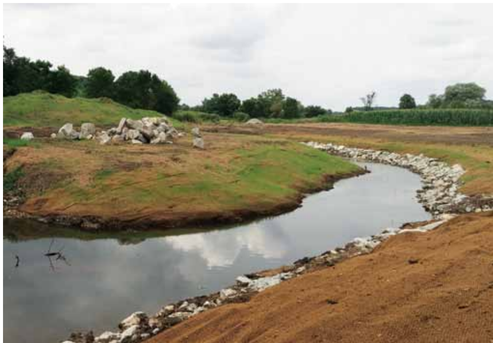
GENTLY SLOPED BANKS ARE SEEDED AND COVERED IN EROSION CONTROL FABRIC AFTER INITIAL GRADING AND CHANNEL WORK IN THE PHOTO ON THE LEFT. A YEAR LATER, NATIVE VEGETATION THRIVES IN AUGUST OF 2016 AFTER COMPLETED RESTORATION WORK ON MILL CREEK IN THE PHOTO ON THE RIGHT.
