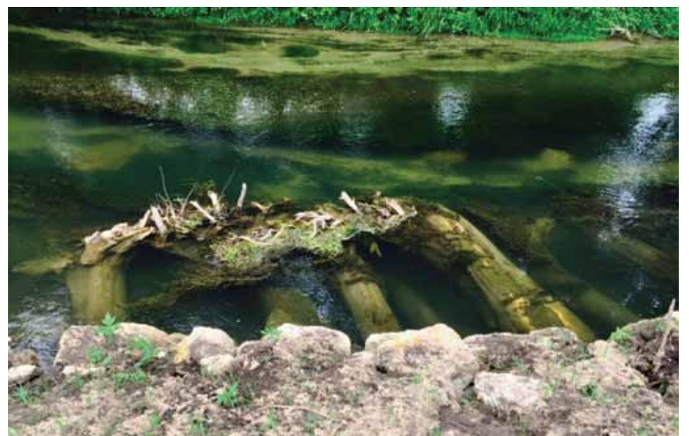
A SECTION OF TROUT COVER INSTALLED ON RUSH CREEK IN SE MN BY THE DNR FISHERIES CREW FROM LANESBORO, MN
