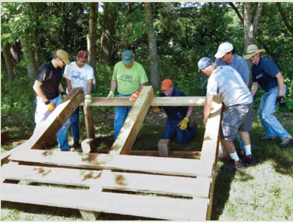
TCTU VOLUNTEERS BUILDING SKYHOOK STRUCTURES FOR USE ON HAY CREEK
