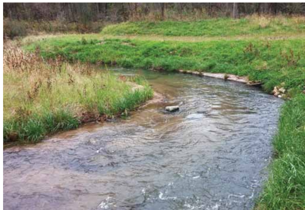
HAY CREEK - AFTER: THE STREAM HAS BEEN SHIFTED AWAY FROM HIGH BANKS. A LOW TERRACE (FLOODPLAIN) HAS BEEN CREATED ALONG WITH DEEP POOLS AND UNDERCUT BANKS. THE GRAVEL AND COBBLE BOTTOM HAS BEEN EXPOSED, IMPROVING INVERTEBRATE HABITAT AND TROUT SPAWNING AREAS.
