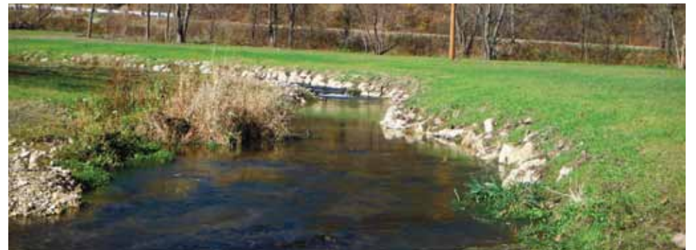
RECENTLY COMPLETED WIN-CRES HABITAT IMPROVEMENT ON GARVIN BROOK
