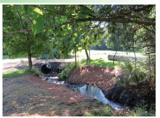
MATUSKA'S CREEK NEAR GRAND RAPIDS MINNESOTA AFTER THE RECENT CULVERT REPLACEMENT. NOTE THE DRY CULVERT ON THE LEFT DESIGNED TO HANDLE HIGH FLOW EVENTS.
