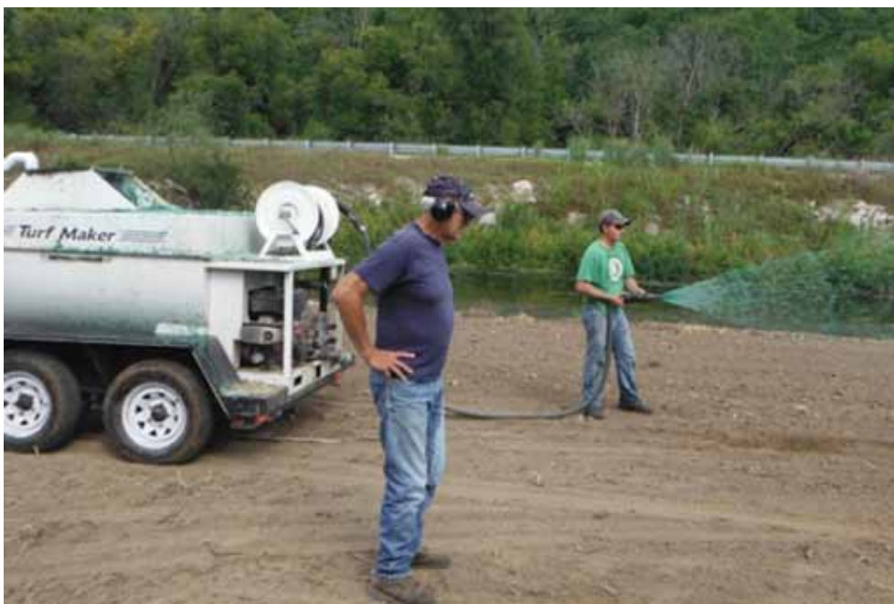
THE FINAL STEPS OF RESEEDING THE GARVIN BROOK PROJECT AREA AFTER A LONG SUMMER OF WORK NEAR WINONA, MN
