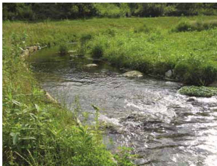
AFTER: BANKS STABILIZED AND RESLOPED
