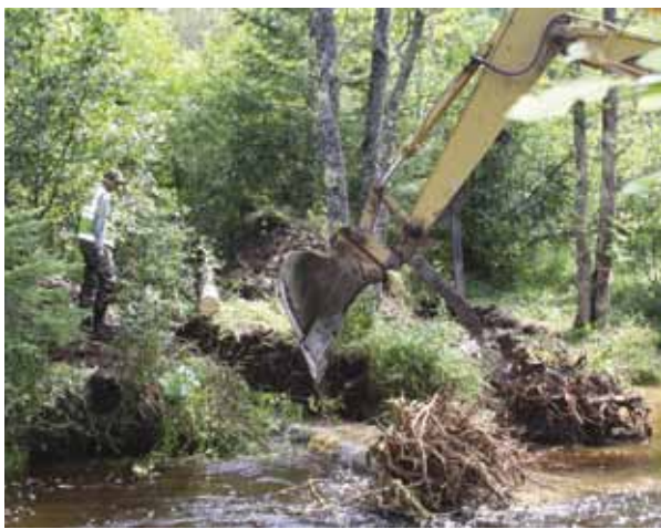
LOGS BEING PLACED AND ANCHORED INTO BANK
