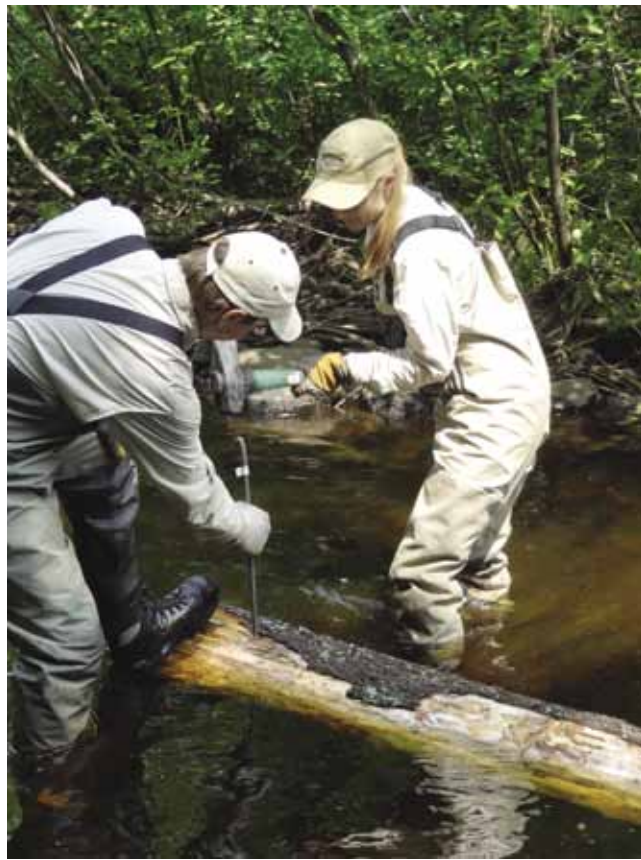
INSTALLING A HALF-LOG IN THE LITTLE ISABELLA RIVER
