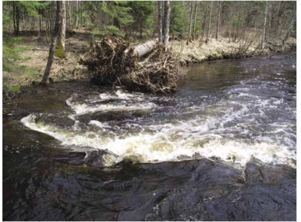
ROCK WEIR CREATING DEEP SCOUR POOL
