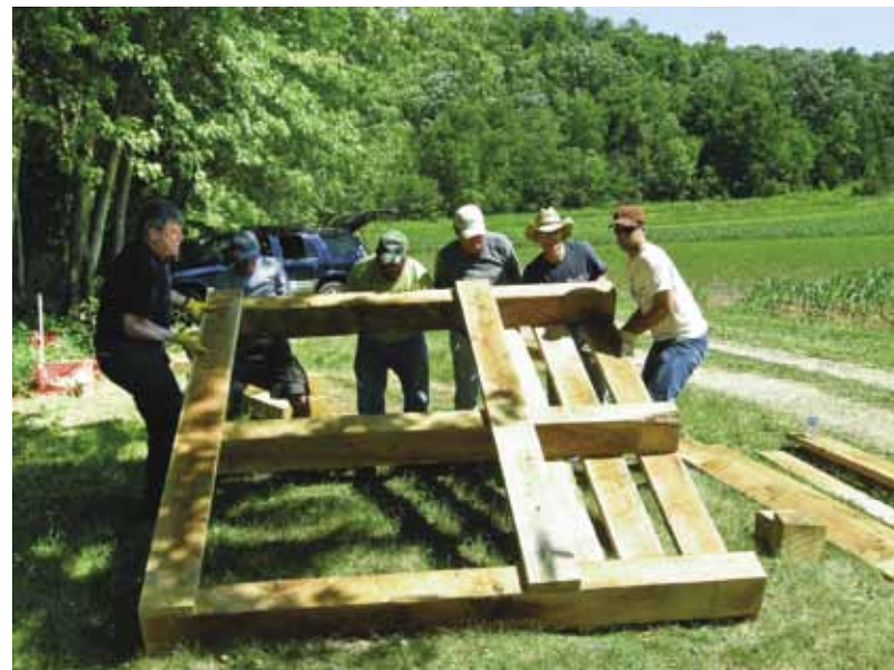
PREPARING A LUNKER STRUCTURE FOR PLACEMENT IN HAY CREEK.
